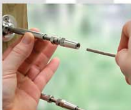
Step 1 Fully seat wire rope.
