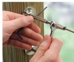
Step 3 Rotate body to tension wire rope.
