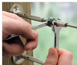
Step 2 Tighten cone onto receiver.
